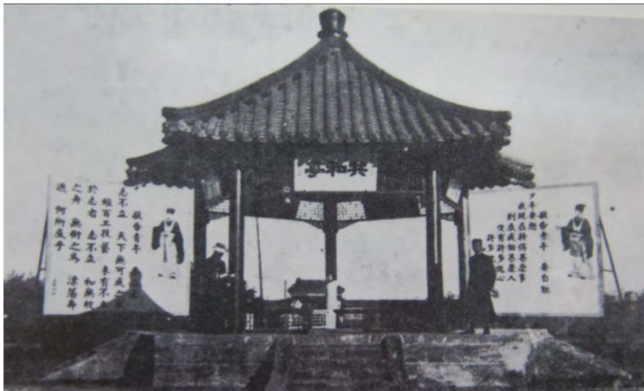
Fig. 1. Venice Gonghe Pavilion, from Xue, Dubi, ed., Report on Jingzhao Park (京兆公园纪实, Jingzhao Gongyuan Jishi ), Beijing, 1925. photo no.44.
